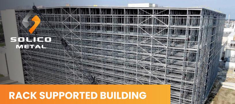
Rack supported structure is comprised of storage systems that act as the structural support for the walls and ceiling of the facility while still providing storage. These can be installed inside, or in addition to, an existing warehouse or designed and built as an exterior structure.
